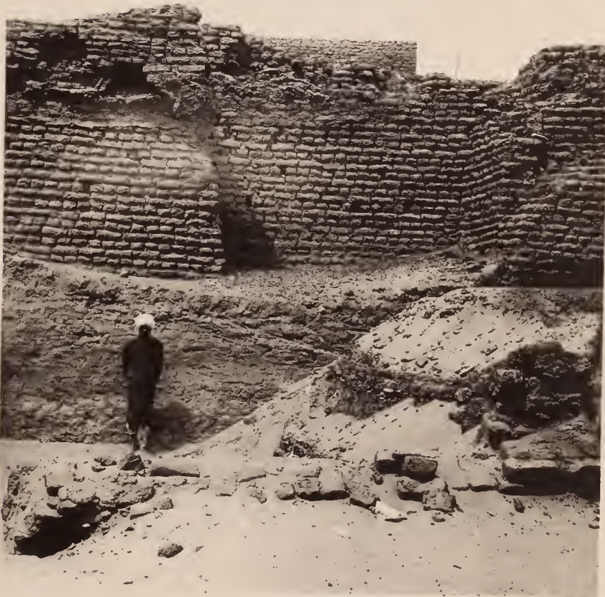
b. Buttress No. 3, to show the height of the wall.
